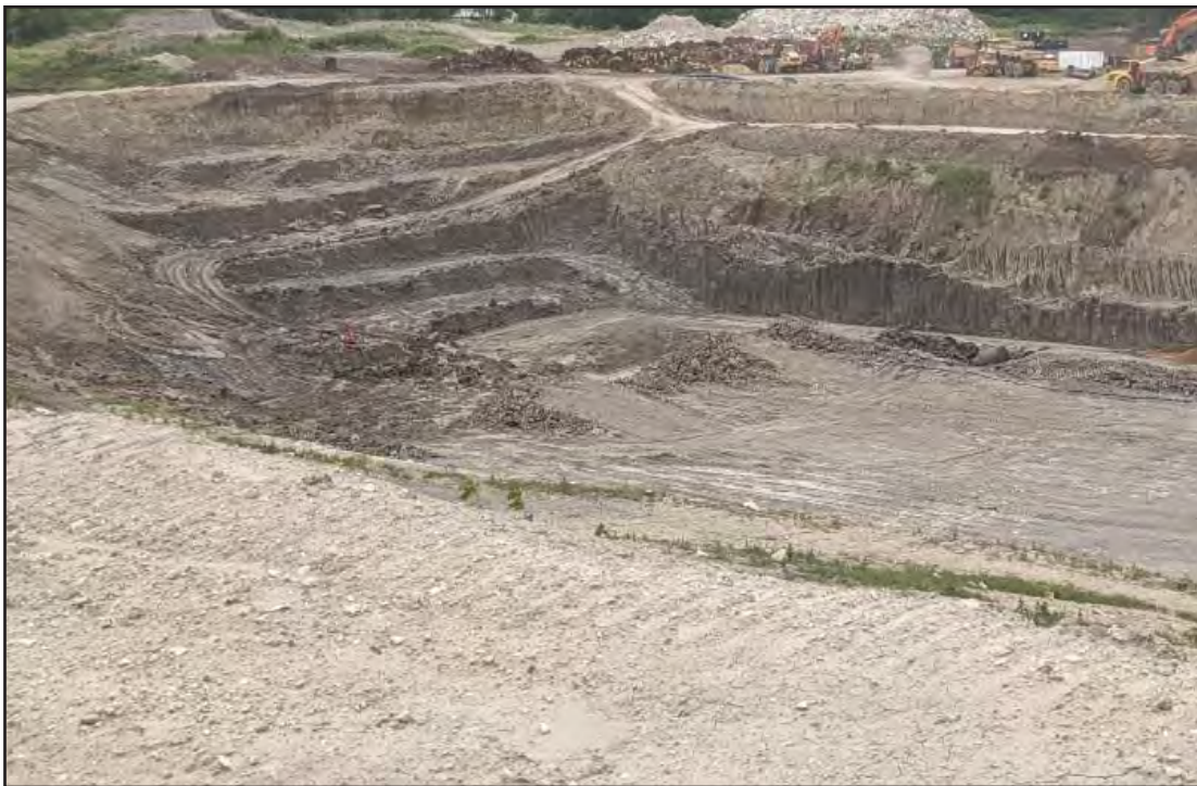
New cell South slope still being shaped
