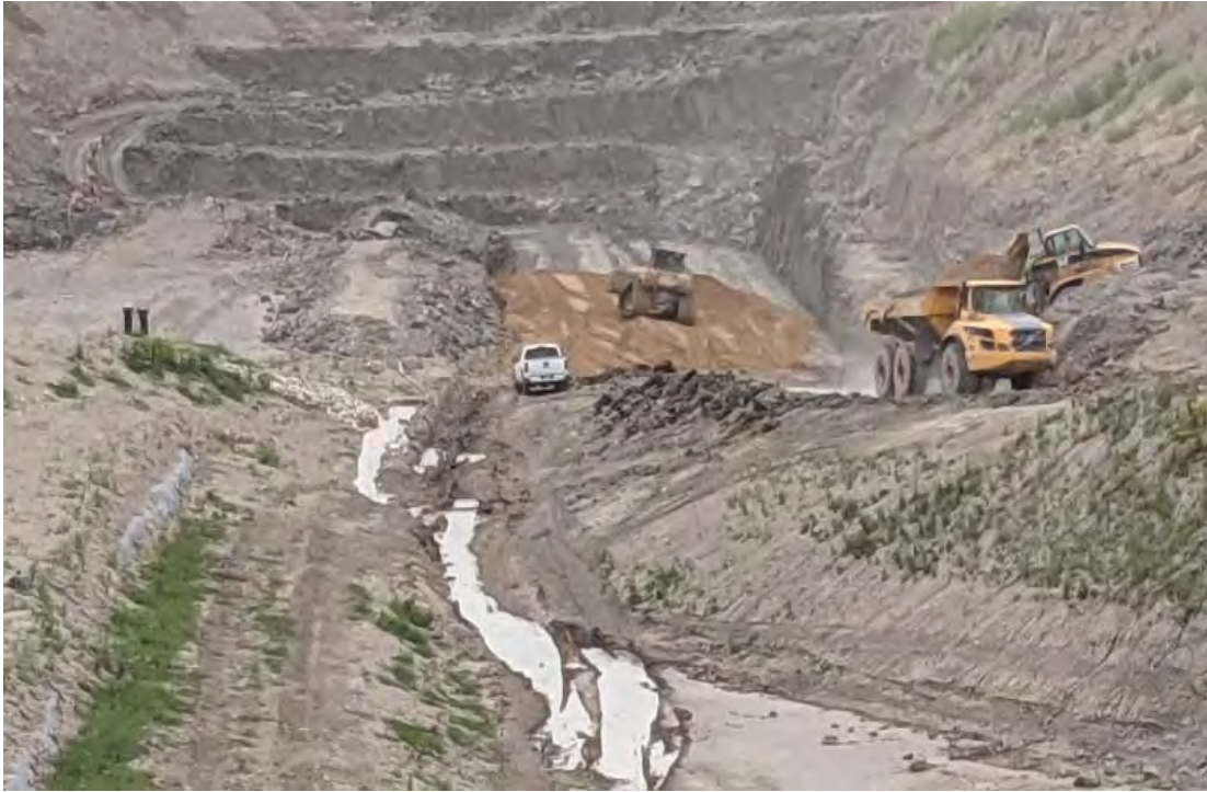
Placement of gradient layer on West side of new cell
