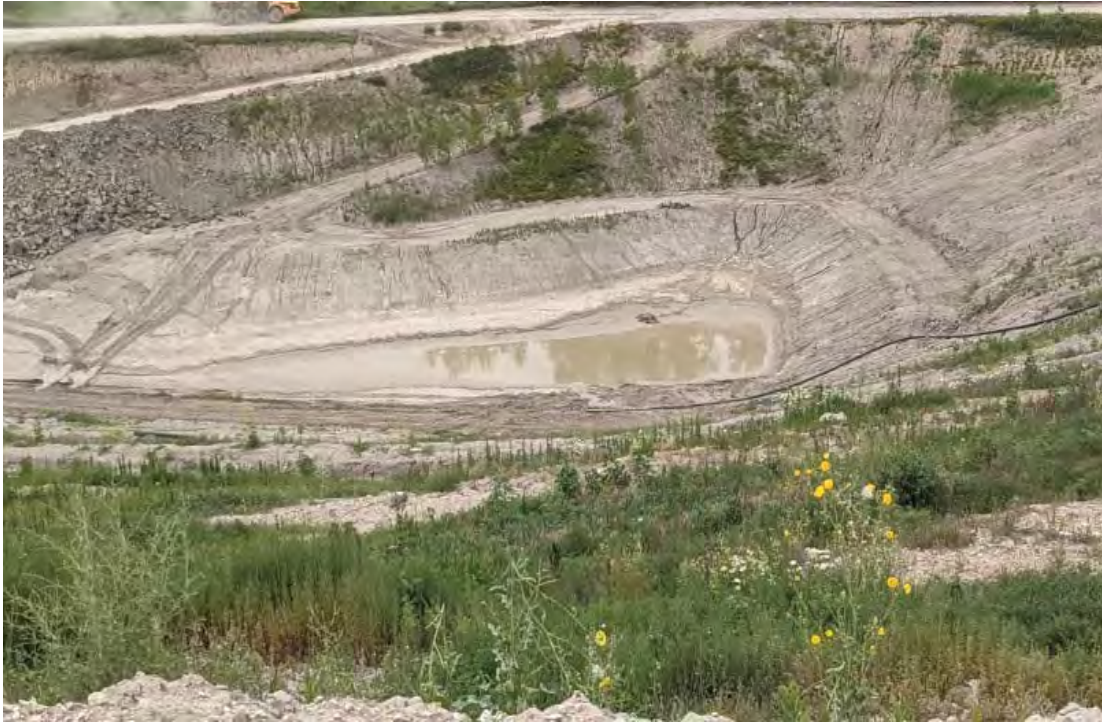
Temp sed basin, being maintained by pumping to Basin #1
