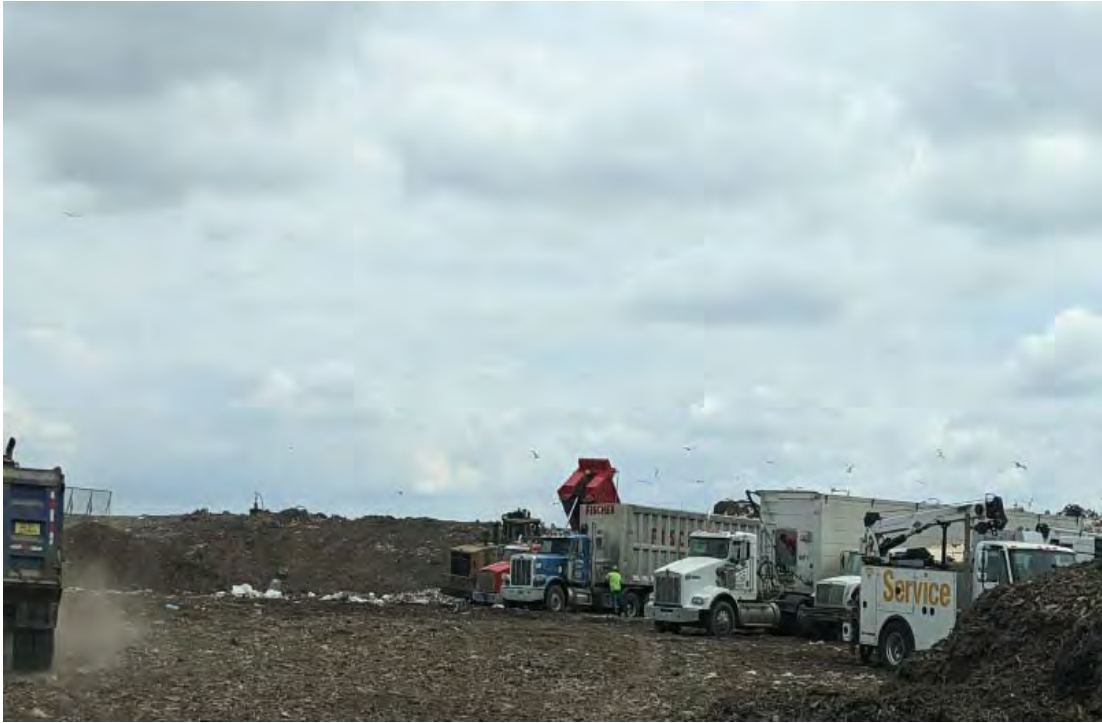
Previously placed waste acting as protective berm about Phase 6. Cover is autofluff ADC
