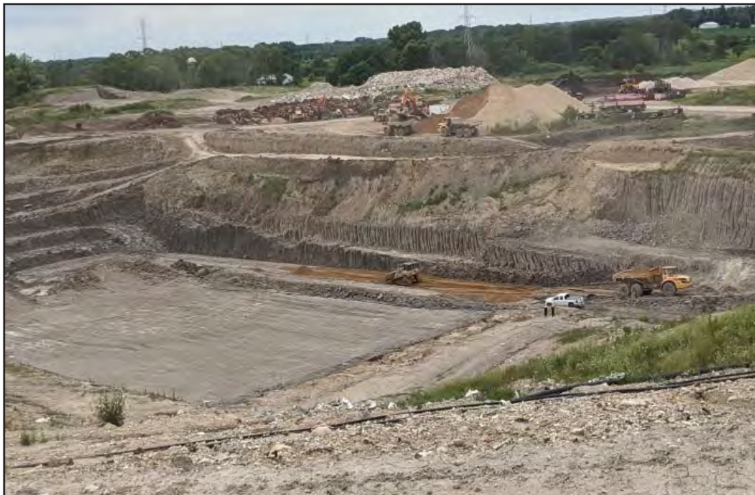
Overview of new cell construction
