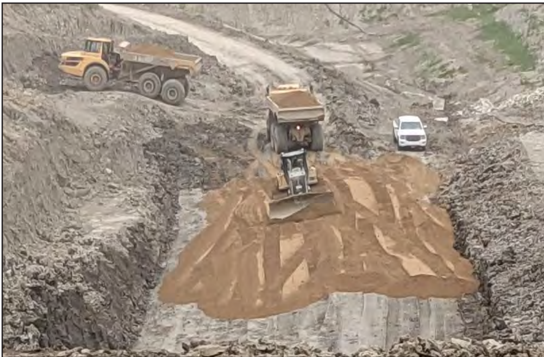
Placement of gradient layer below liner in new cell
