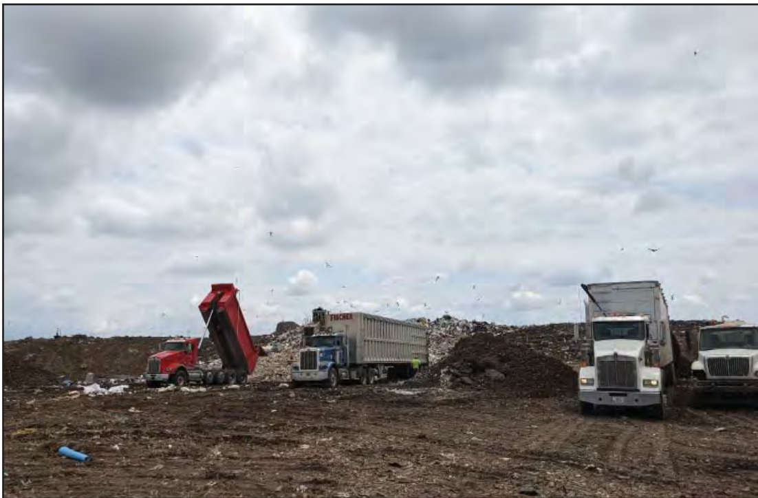
Working face moving along South end of Phases 6/7
