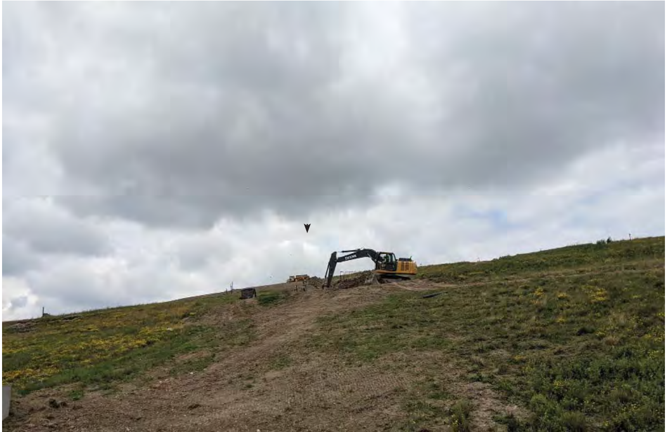
Contractor digging trenches for placement of gas collection piping
