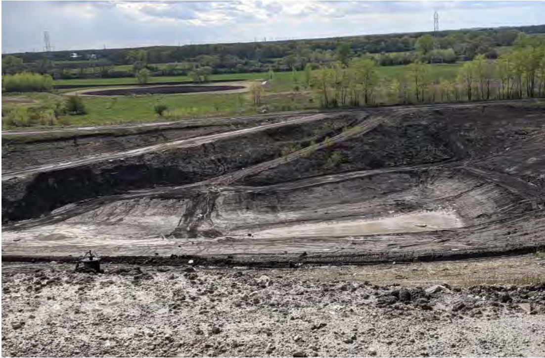
Temp sed basin viewed from the East
