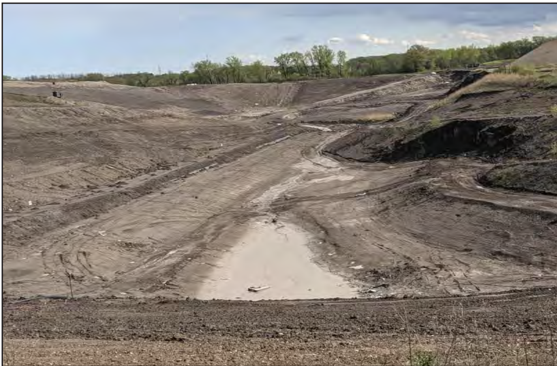
Temp sed basin, maintained in a dry condition
