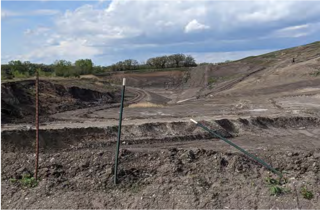
Temp sed basin viewed from the South
