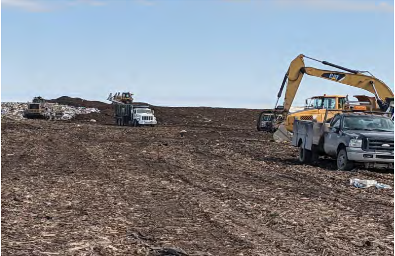
Previous working faces to the South of current, creating protective berm about lip of Phase 7
