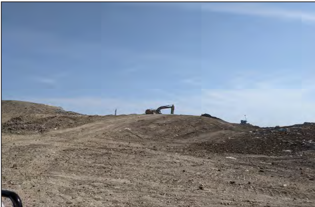
West side of bio pile being excavated for treatment
