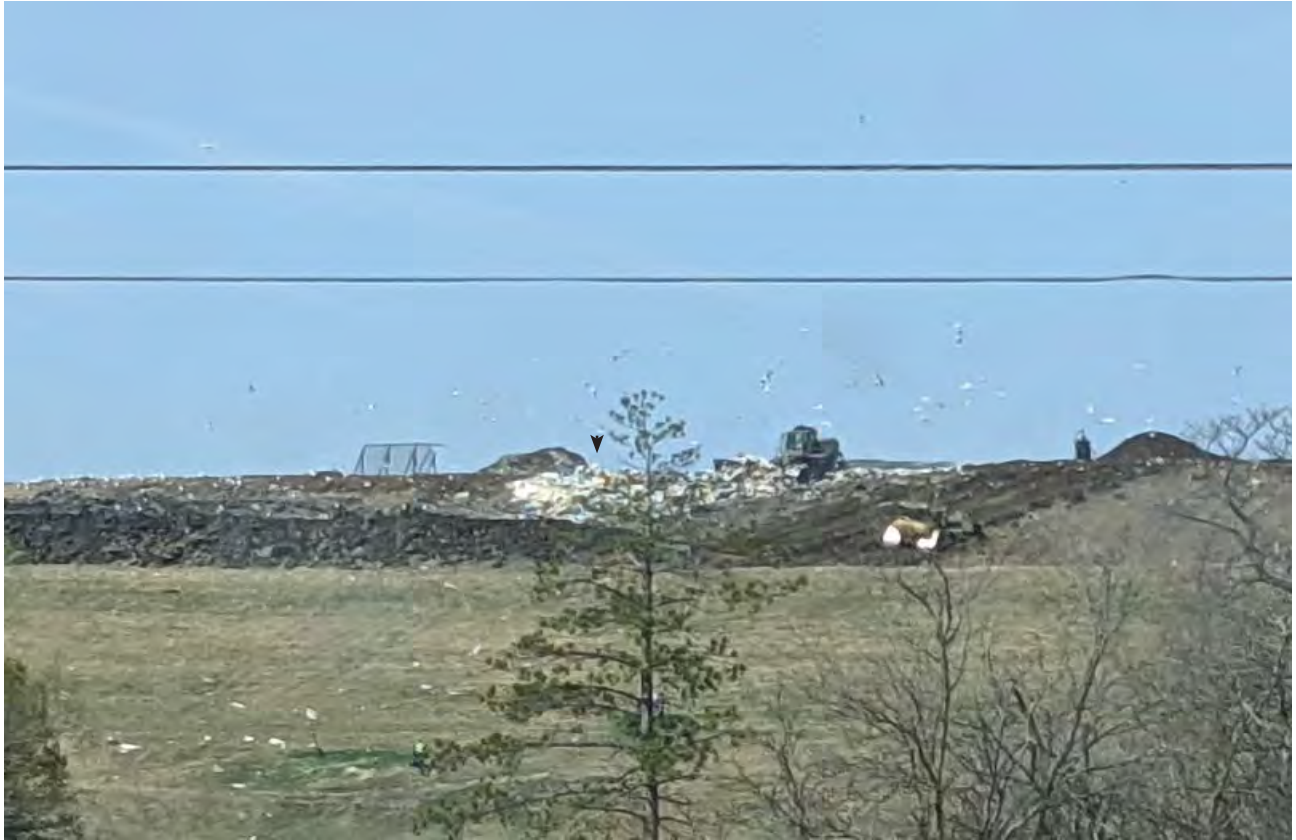
Working face in Phase 6, East slope
