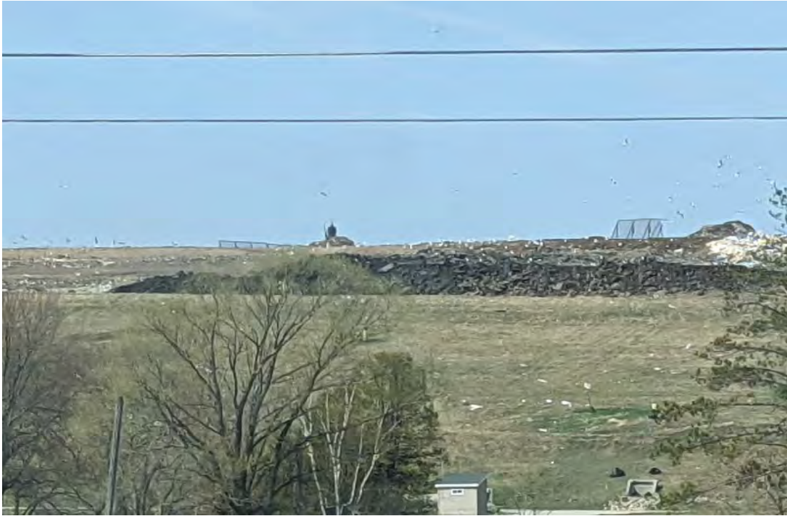
Soil being pulled back for future waste placement
