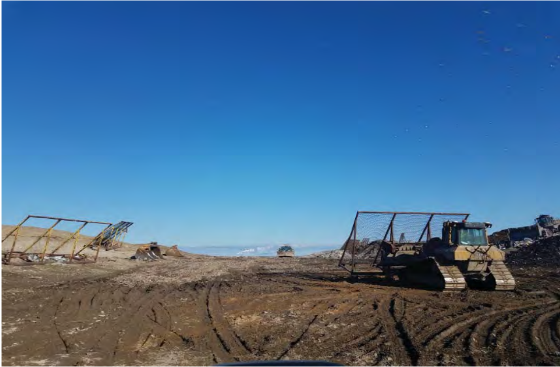
Fence actively being relocated for litter control
