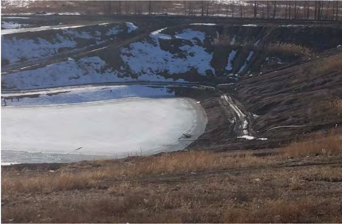
Temp sed basin, pump placed in thawed water
