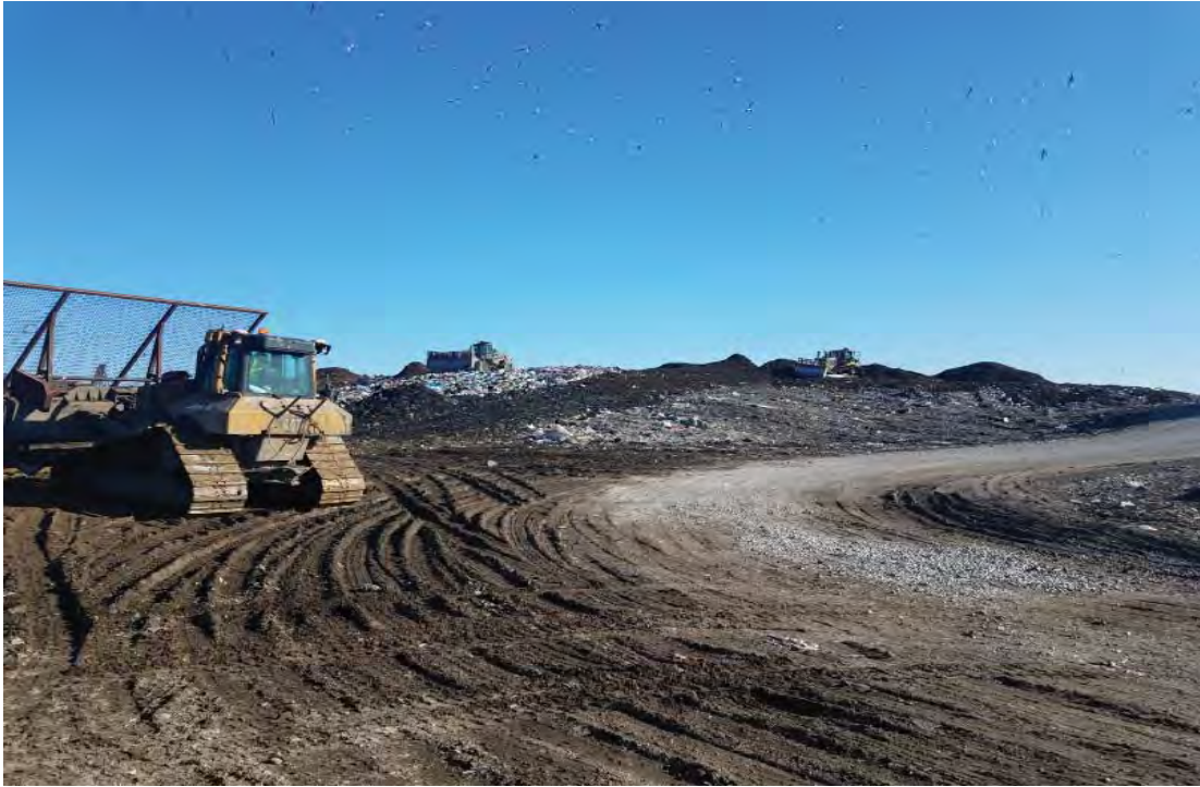
Access to active area
