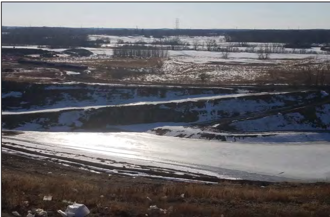
Temp sed basin beginning to thaw, pump is in place
