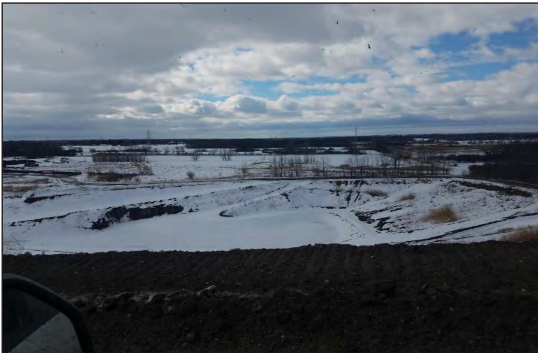
East of Phase 7, temp sed basin and future cells. Well frozen
