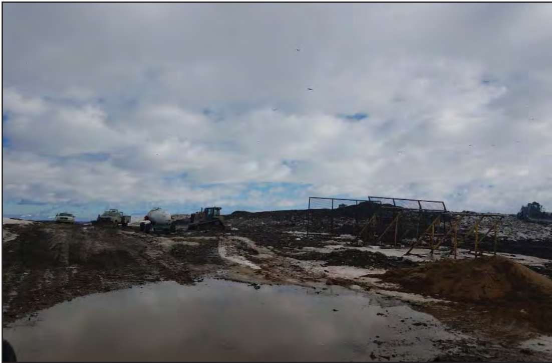
Thawing conditions in Phase 7
