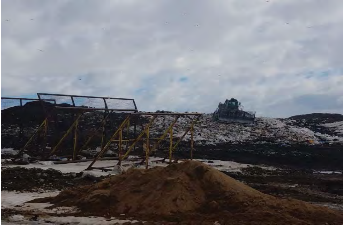
Tipping continues on top of working face and pushing waste down
