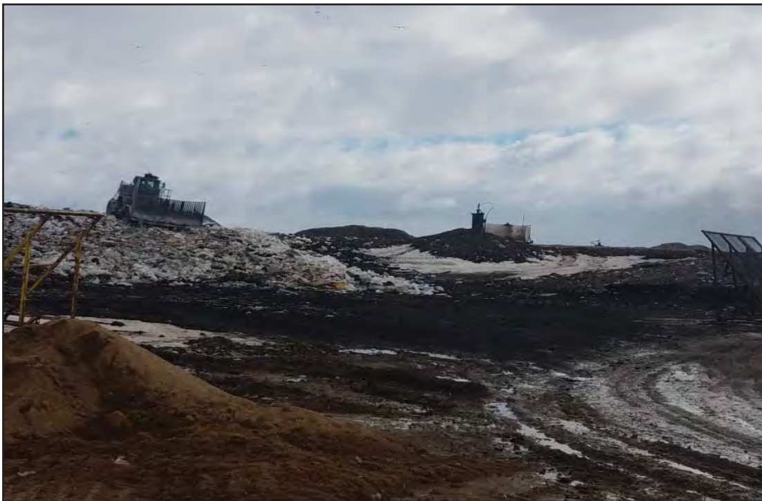
Working face moving Westward across Phase
