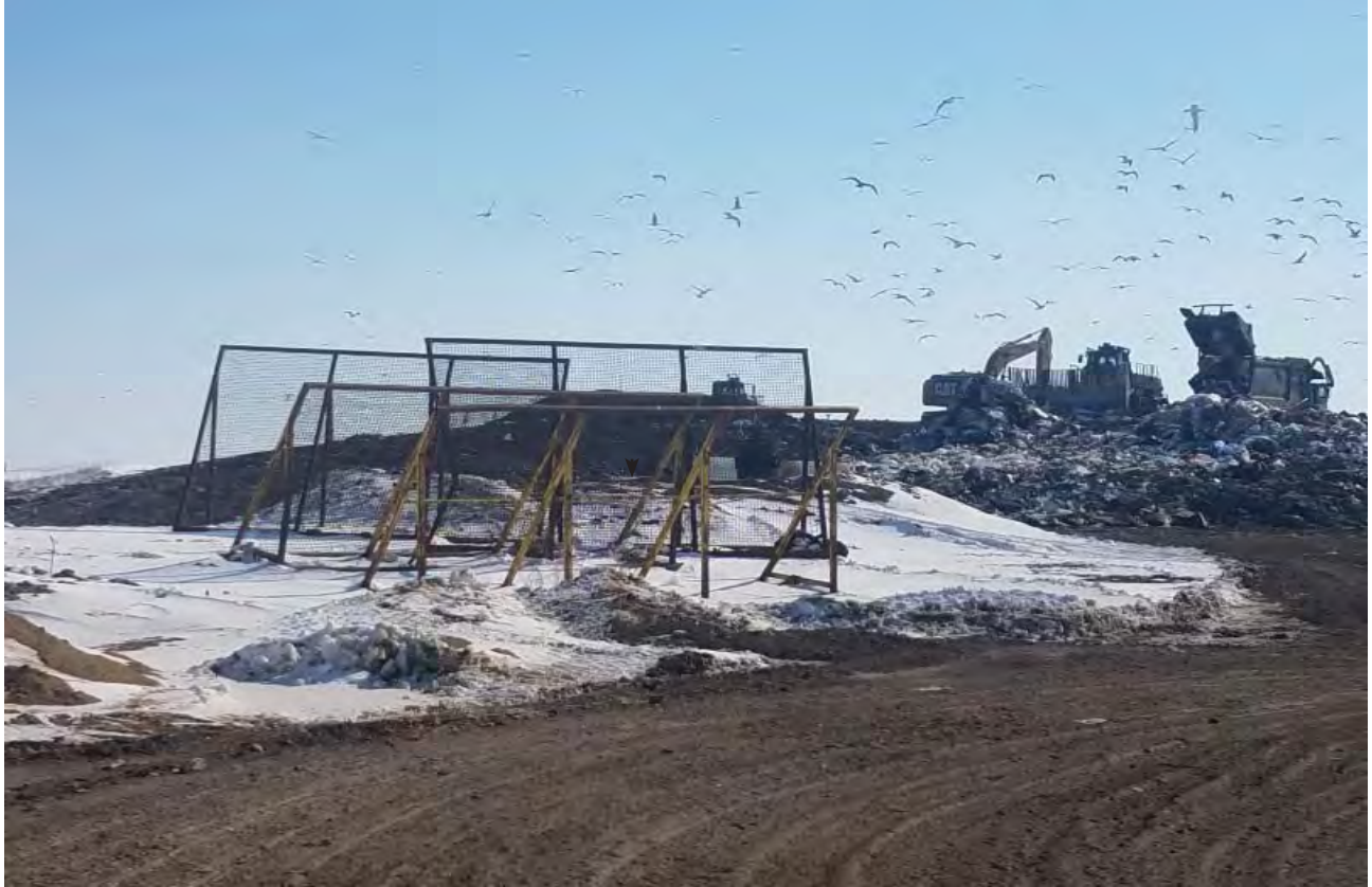
Active area, cleared of snow and receiving waste at top of working face, pushing down with equipment
