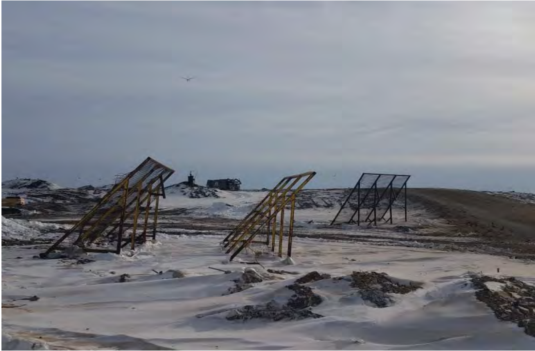
Phase 7, West edge, access road and previous working faces developing a protective berm
