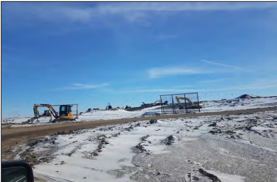
Approach to active area in Phase 7
