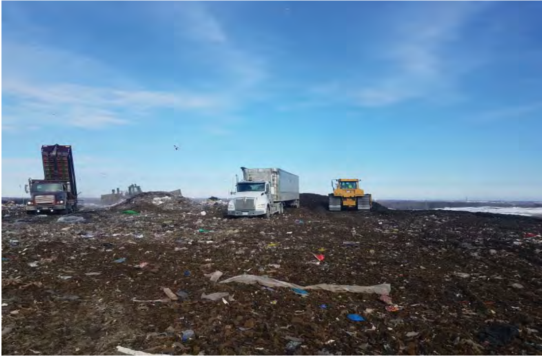
Clean out on Phase 7, dozer spreading cover
