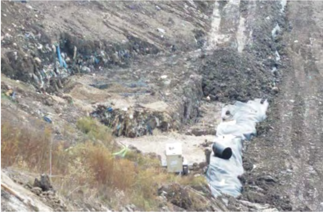
Restored and filled sump in Phase 7
