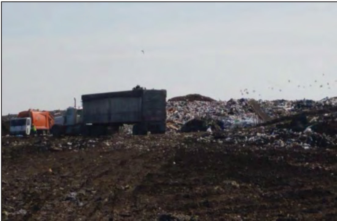
Working face in South end of Phase 7, offset from top of West slope
