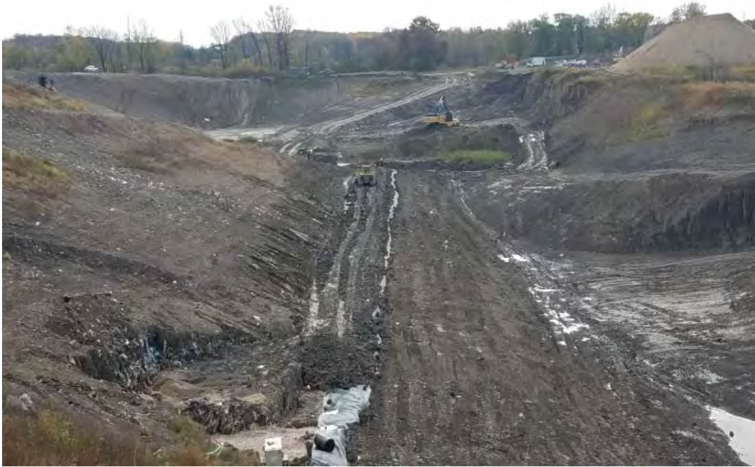
Rainflap repair complete, contractor placing road at base of slope
