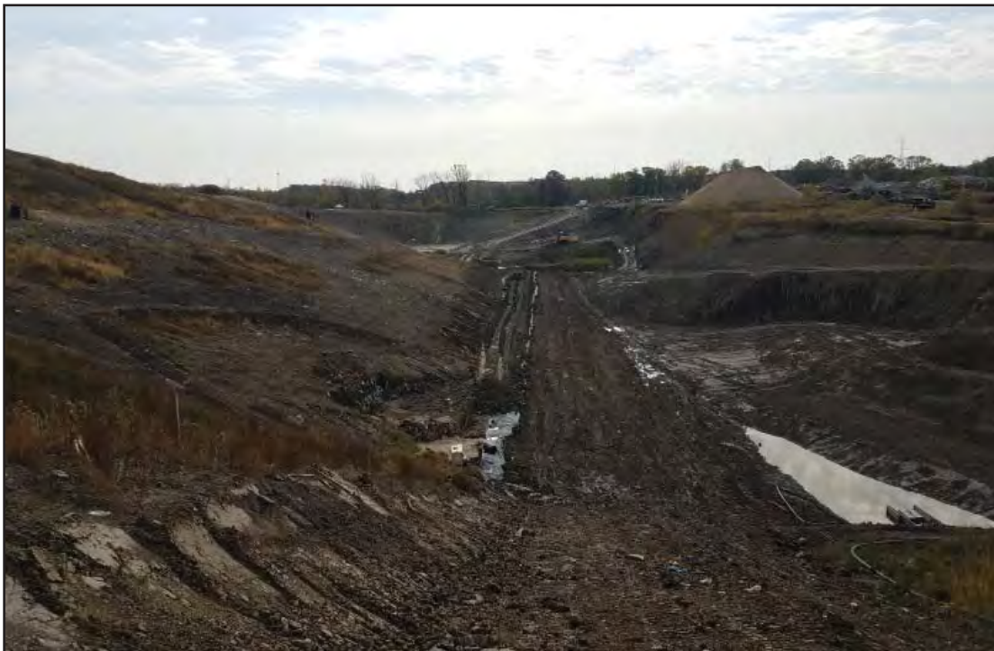
Run of rainflap repaired and temp sed basin regraded
