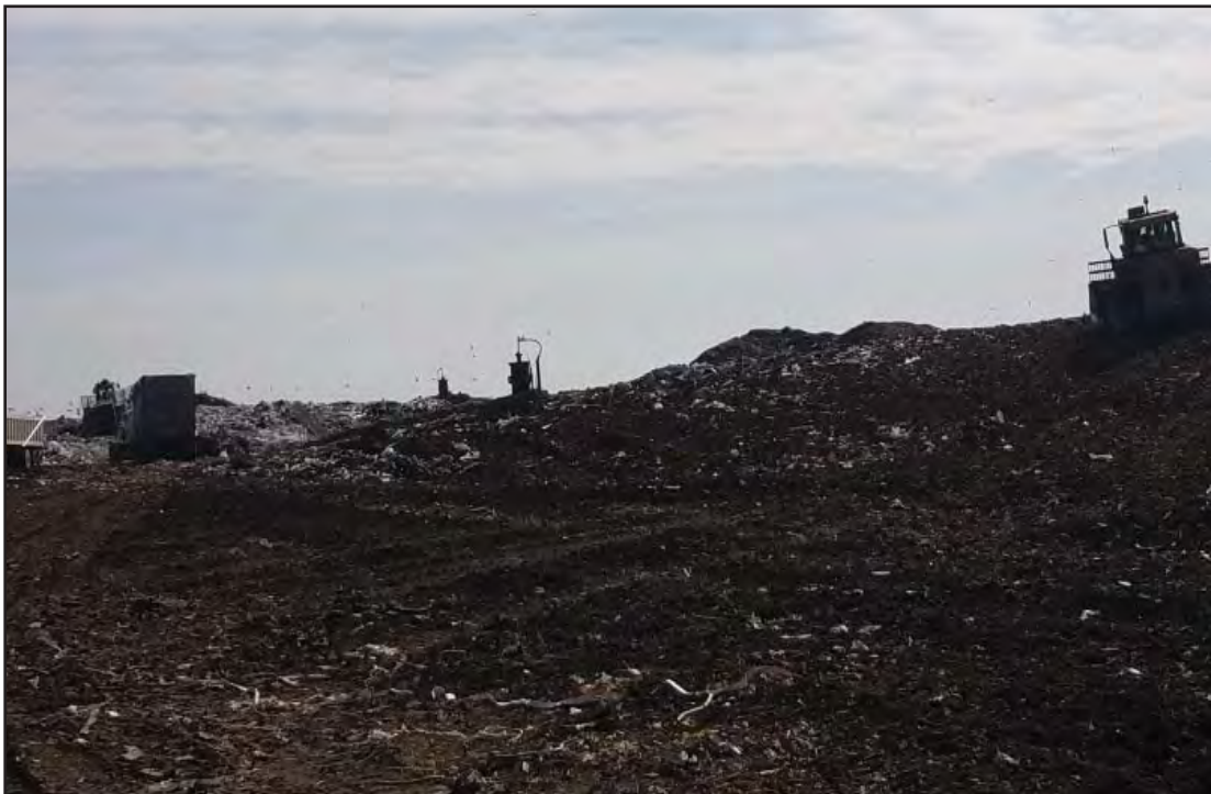
Previous lift along West slope of Phase 7, creates a protected area for current waste placement
