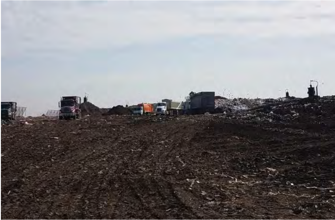
Working face in South end of Phase 7, offset from top of West slope
