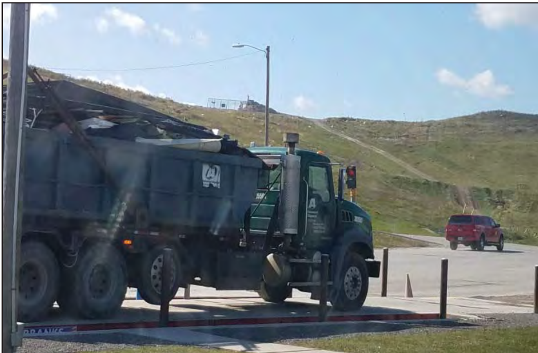
Erosion in Phase 4
