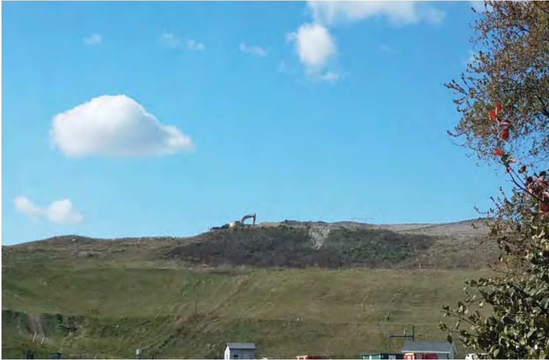
Stockpiled Soils on top of Phase 3
