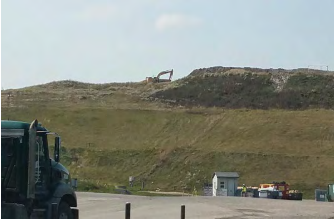
East slope of Phase 1, view of bio and direct soils
