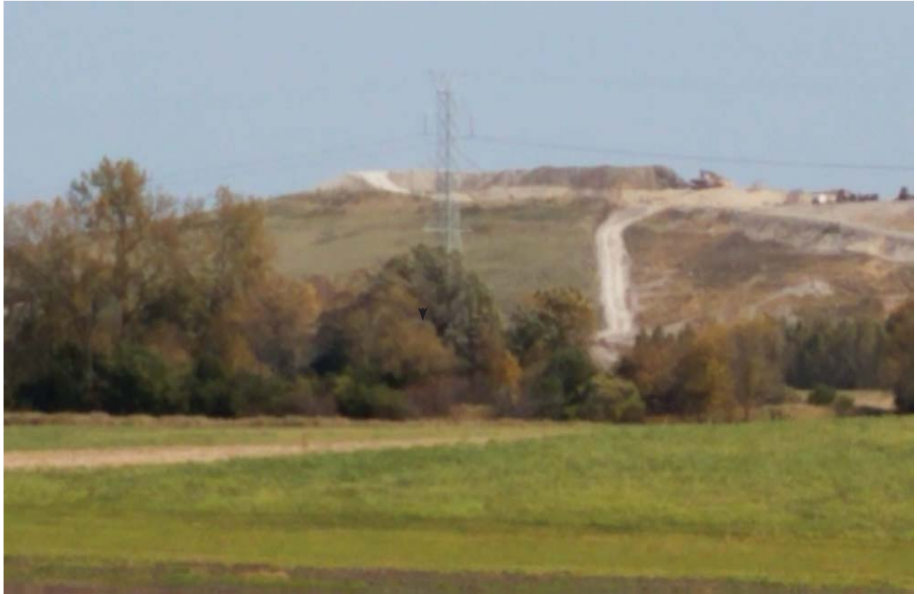
Phase 3, erosion from haul truck activities on West slope
