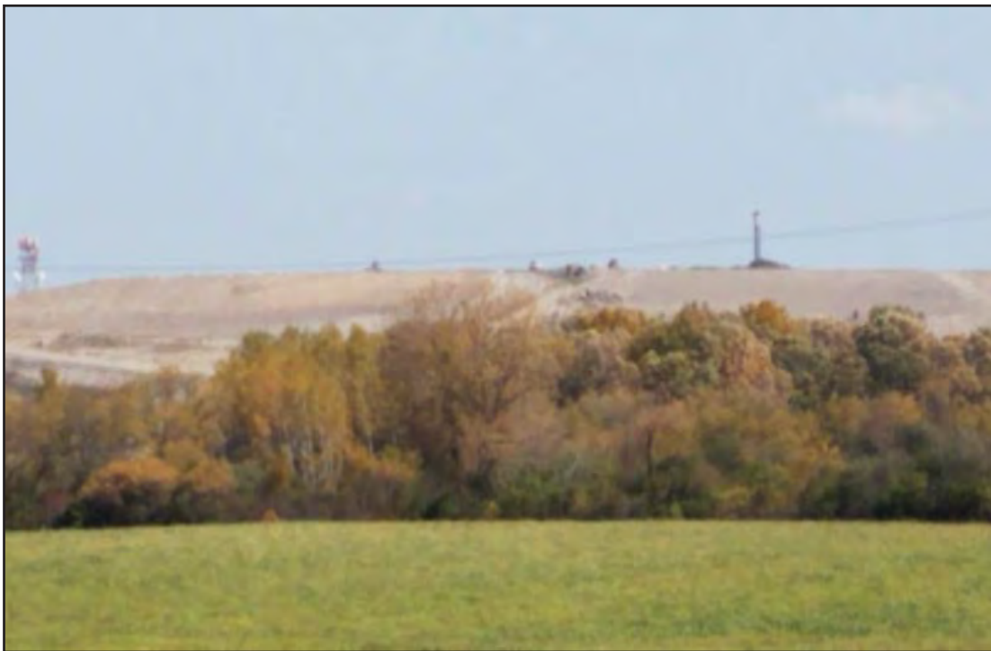
Phase 7 viewed from a distance and the West
