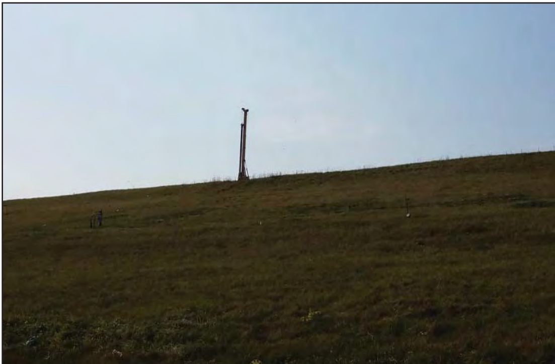
Drill rig in Phase 7 placing replacement gas well
