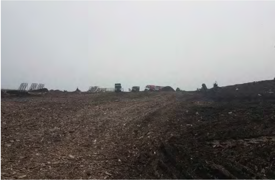
Active area viewed from North, working face below visible grade
