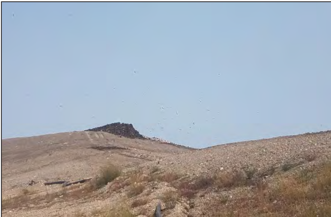
Stockpiled cover adjacent to working face at Southwest corner of Phase 7 South
