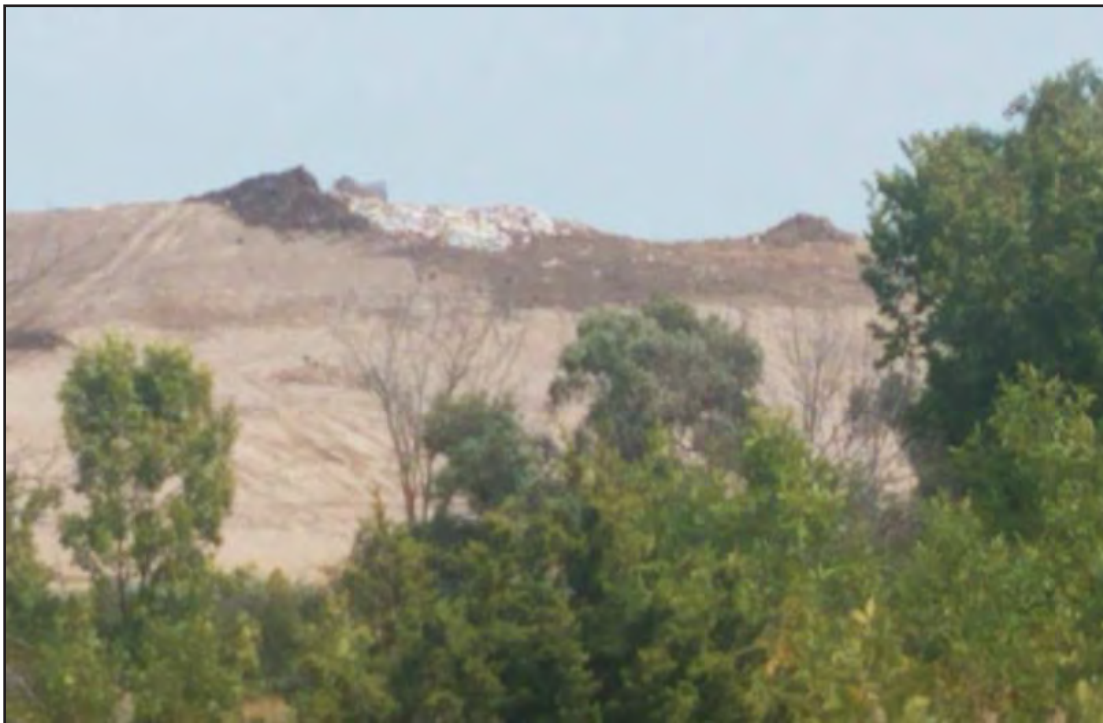
Working face at South end of Phase 7 South
