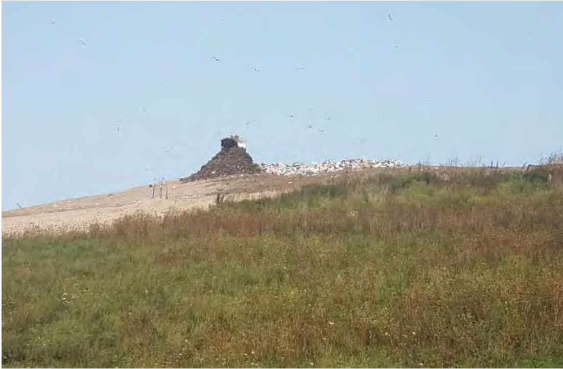
Stockpiled cover adjacent to working face at Southwest corner of Phase 7 South
