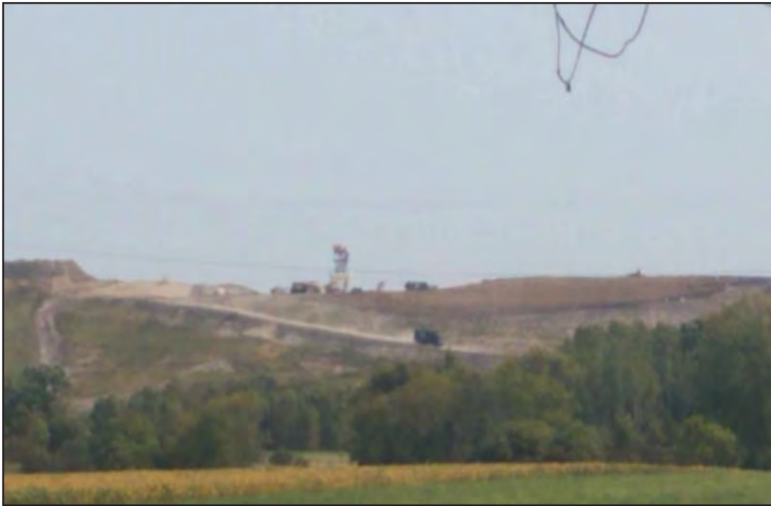
Overview of landfill from West
