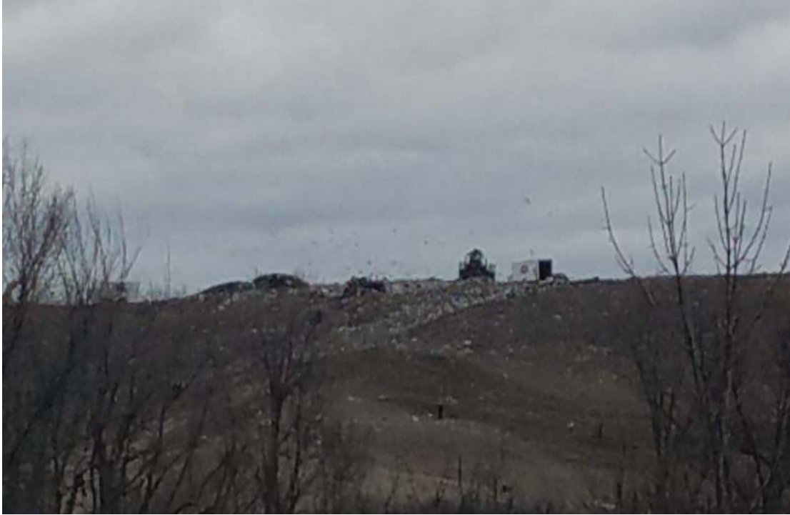
Working face in Phase 7 South viewed from Union Church Road
