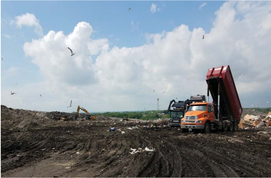
Tipping in Phase 7 South
