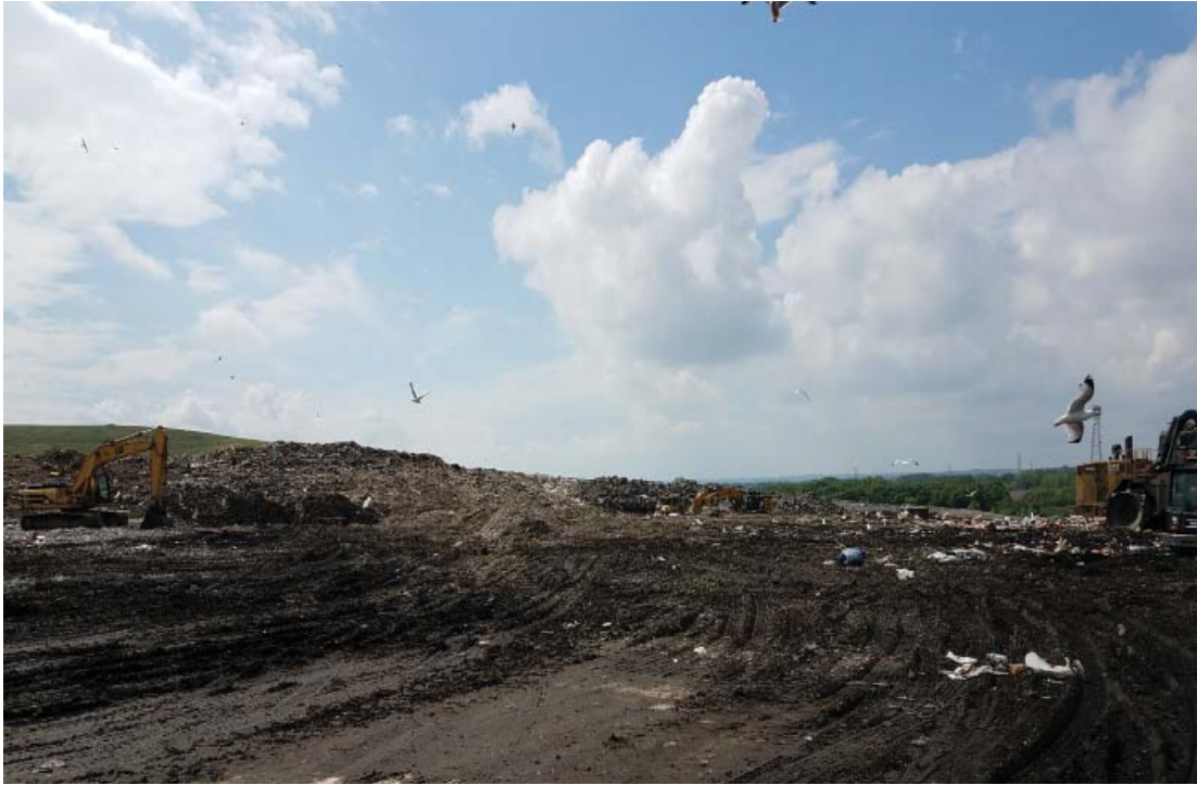
Working face back dragged for better access
