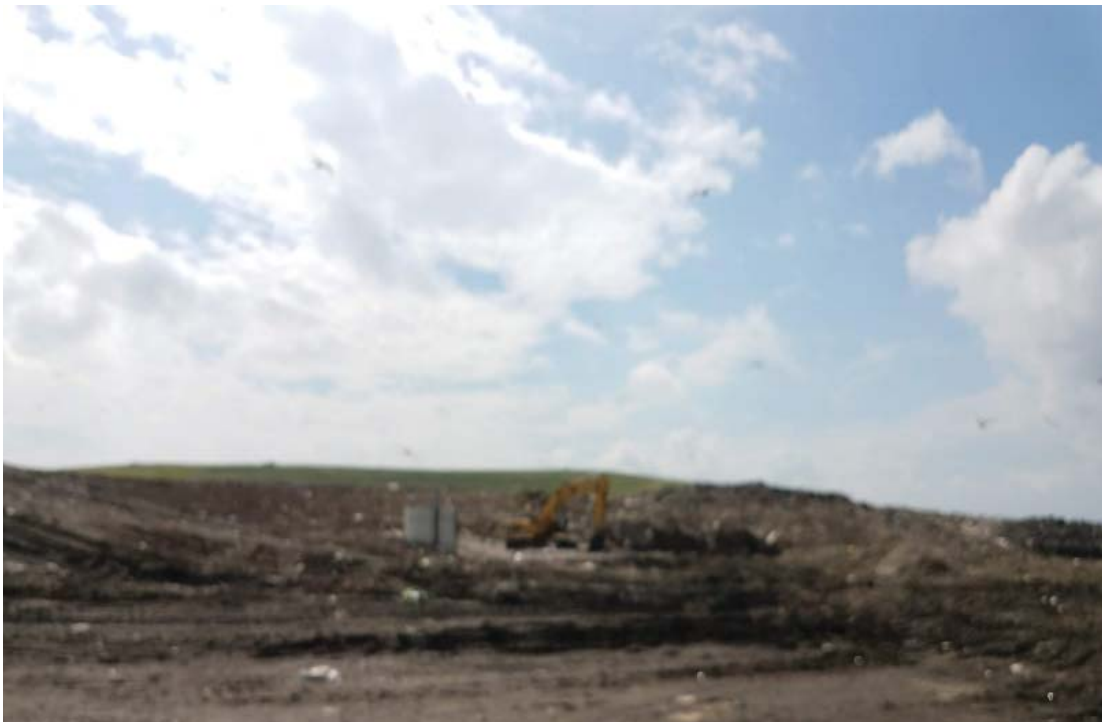
Excavator for clean outs
