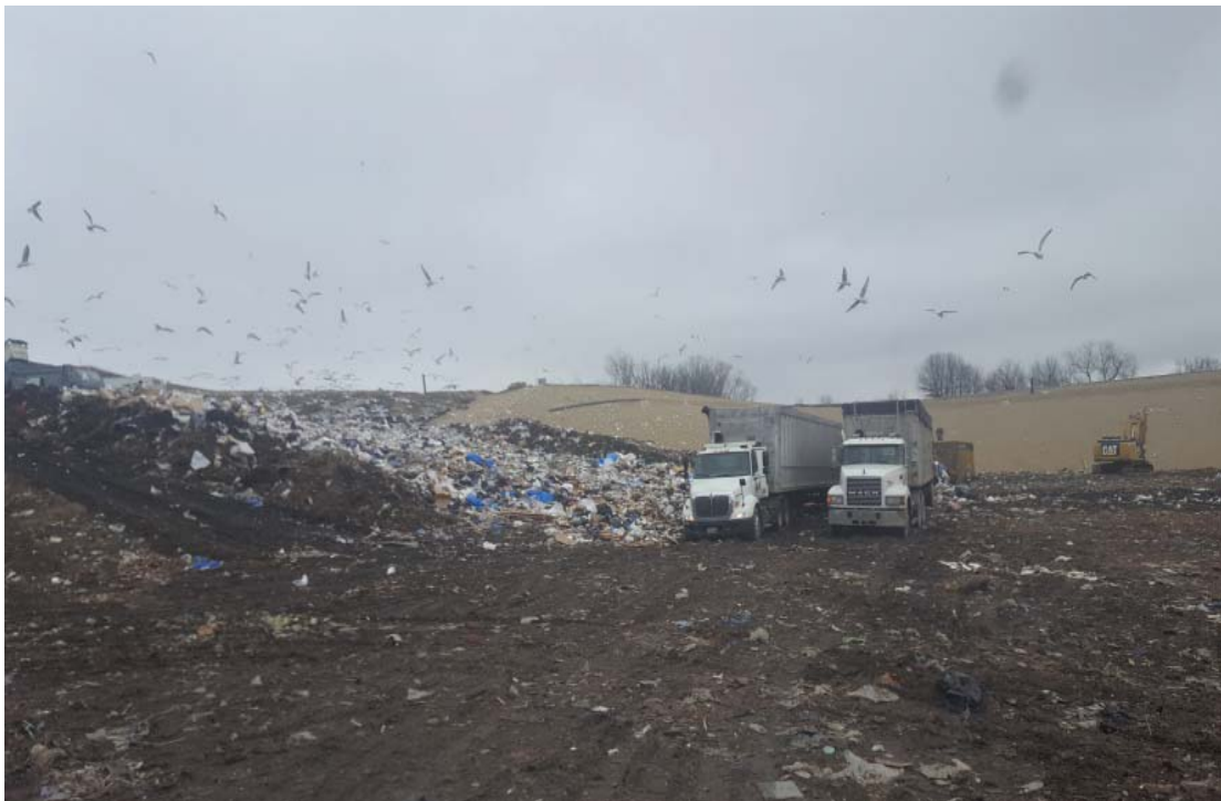
Working face in Phase 7 South, toe of face
