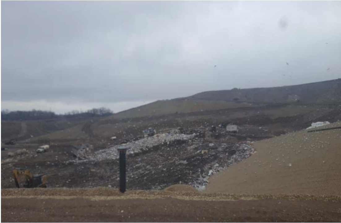
Phase 7 South, working face in center of Phase
