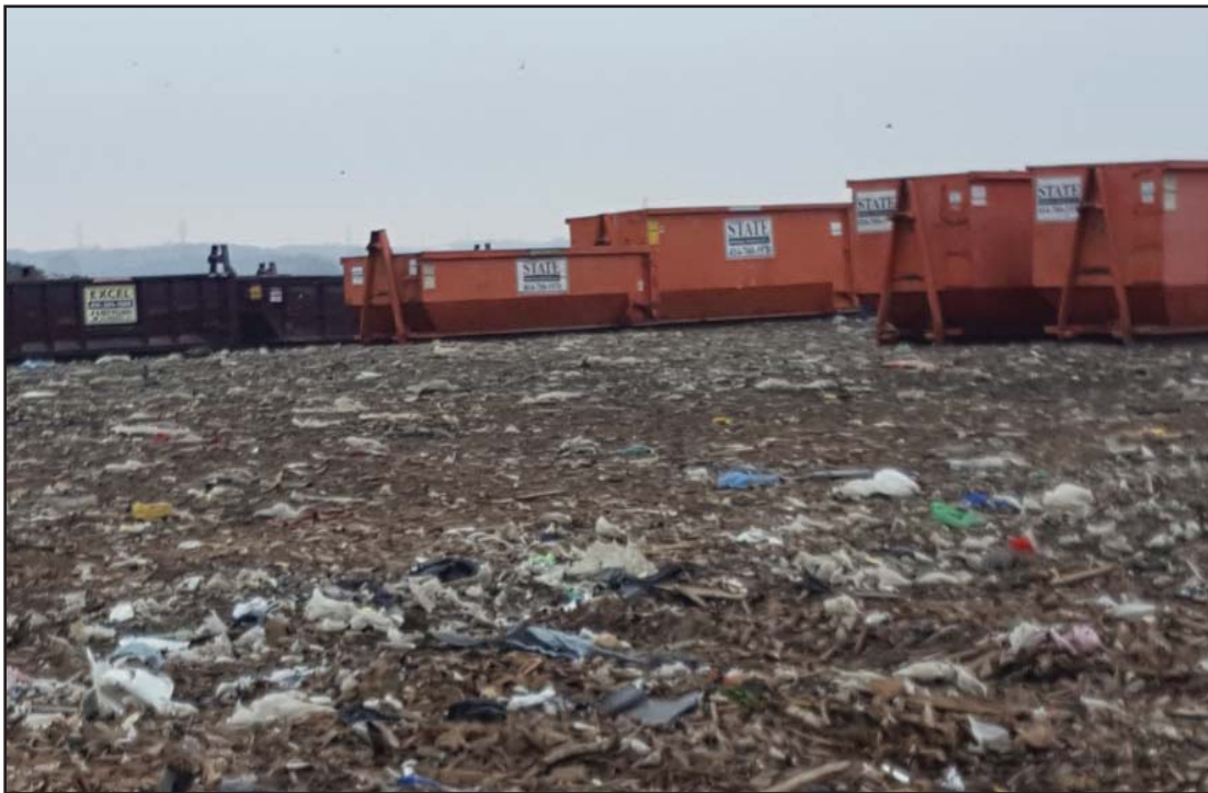
Roll off boxes staged on Phase 7 during road construction.
