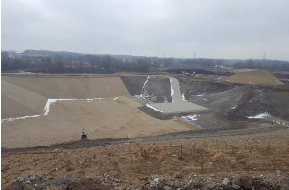
Expansion complete and awaiting DNR approval before waste placement
