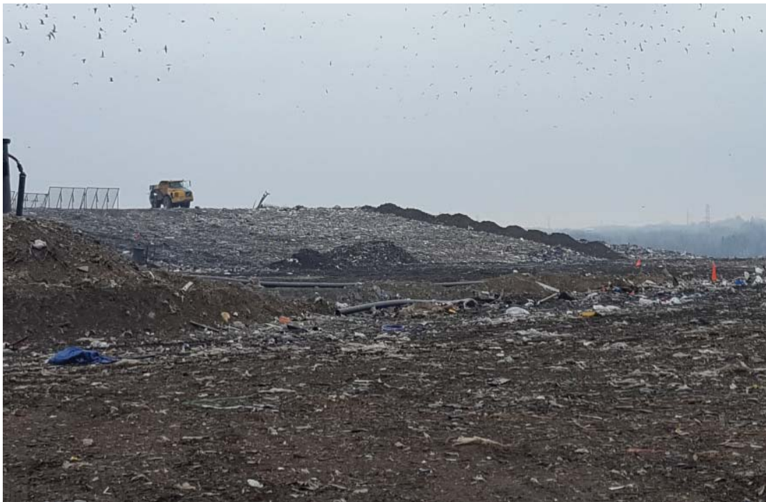
Previous days working face covered with sand and poly-fluff mix (MRF fines)
