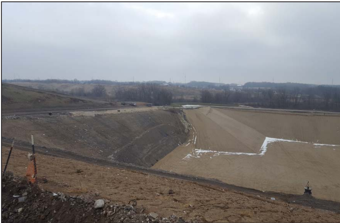
New expansion, East side, awaiting approval prior to waste placement
