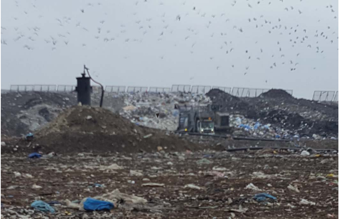
Working face along Phase 6/7 border, note litter fences at top of slope.
