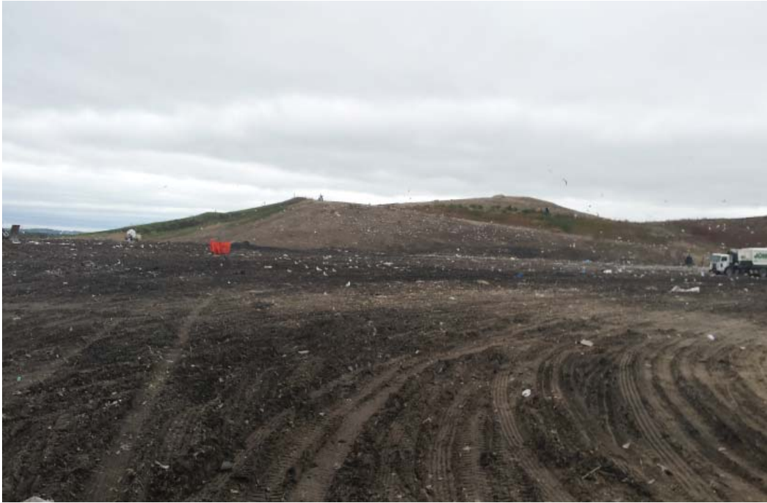
Active area viewed from the across to Phases 1 thru 3
