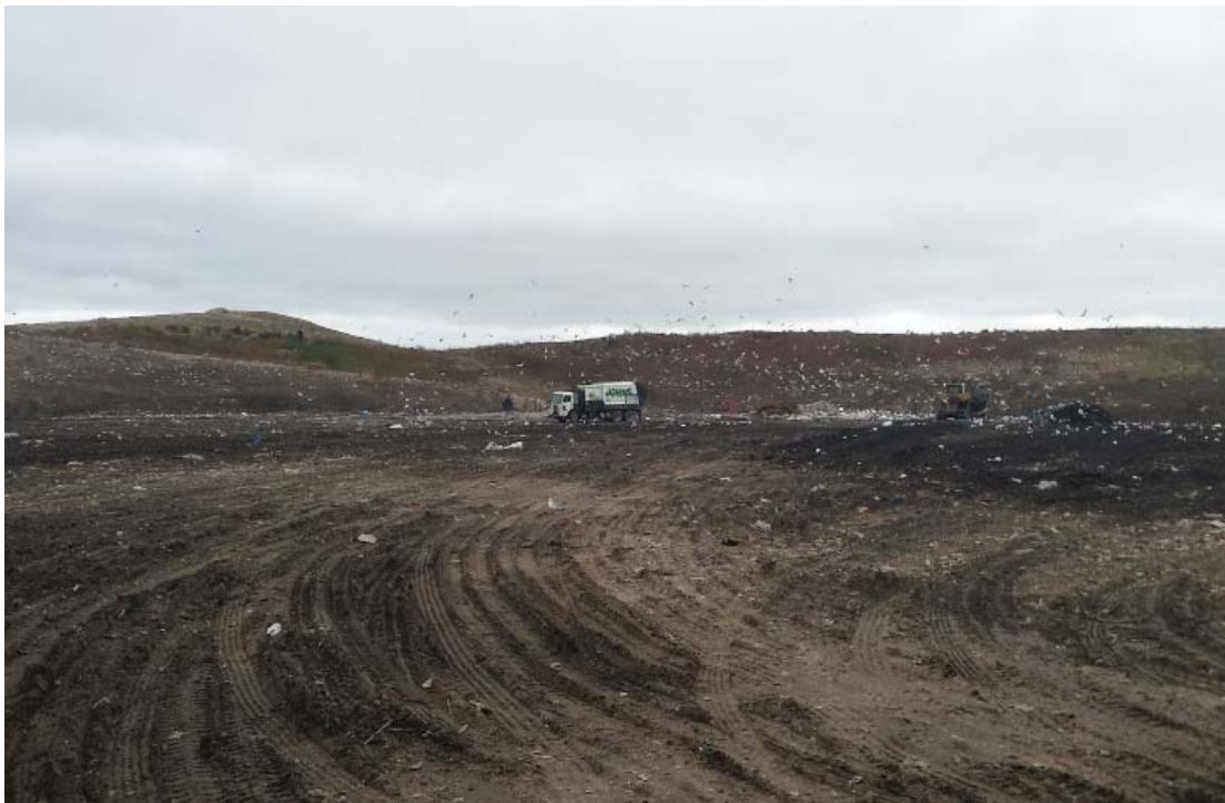
Phase 7 active area viewed from the Southwest corner
