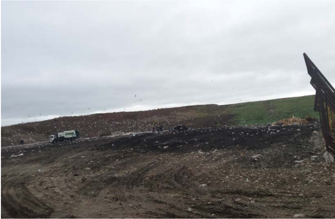
Phase 7 active area viewed from the West
