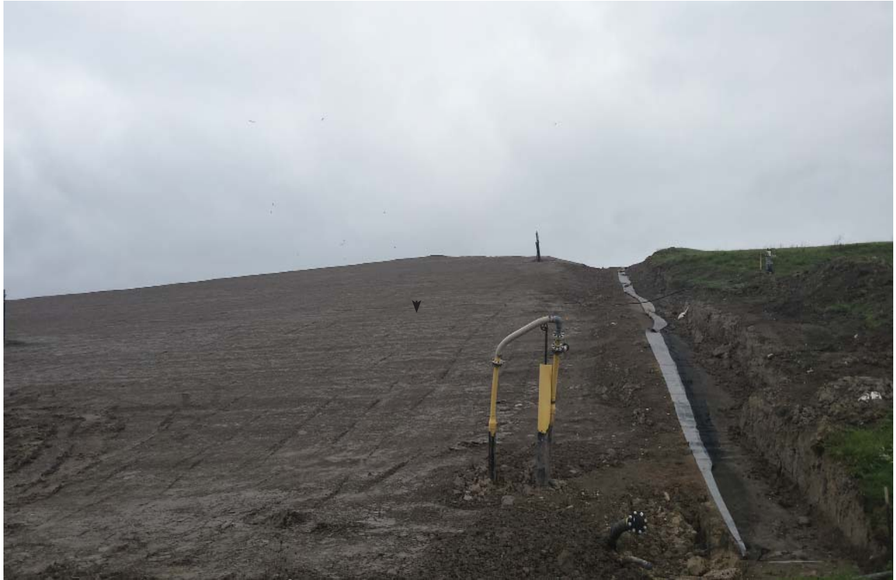
Closure Area IV junction with Closure Area III
