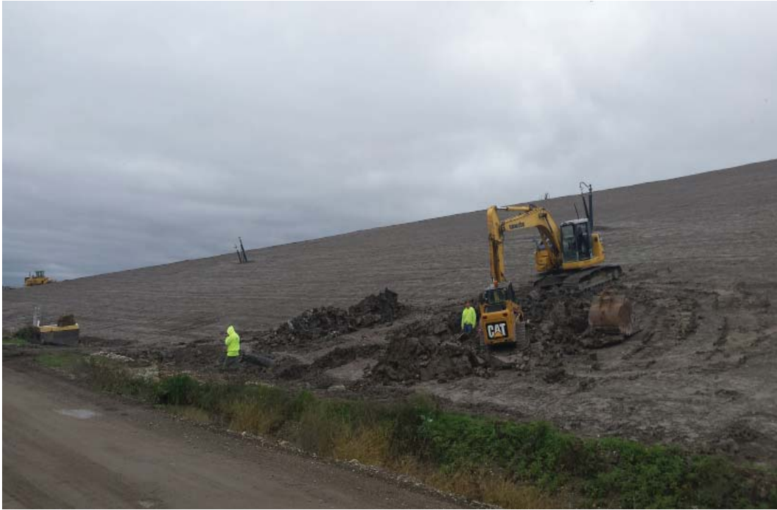
Repair of pneumatic gas line in cover layers
