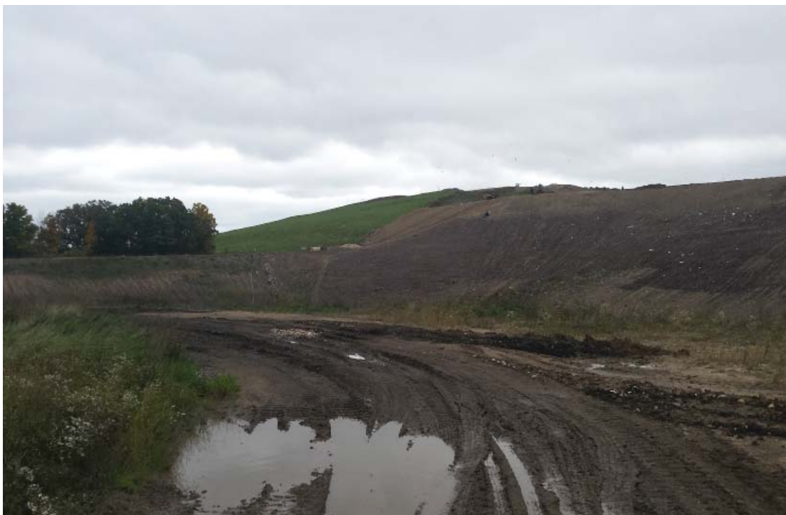
West slope of Phase 7 and slopes of temp sed basin
