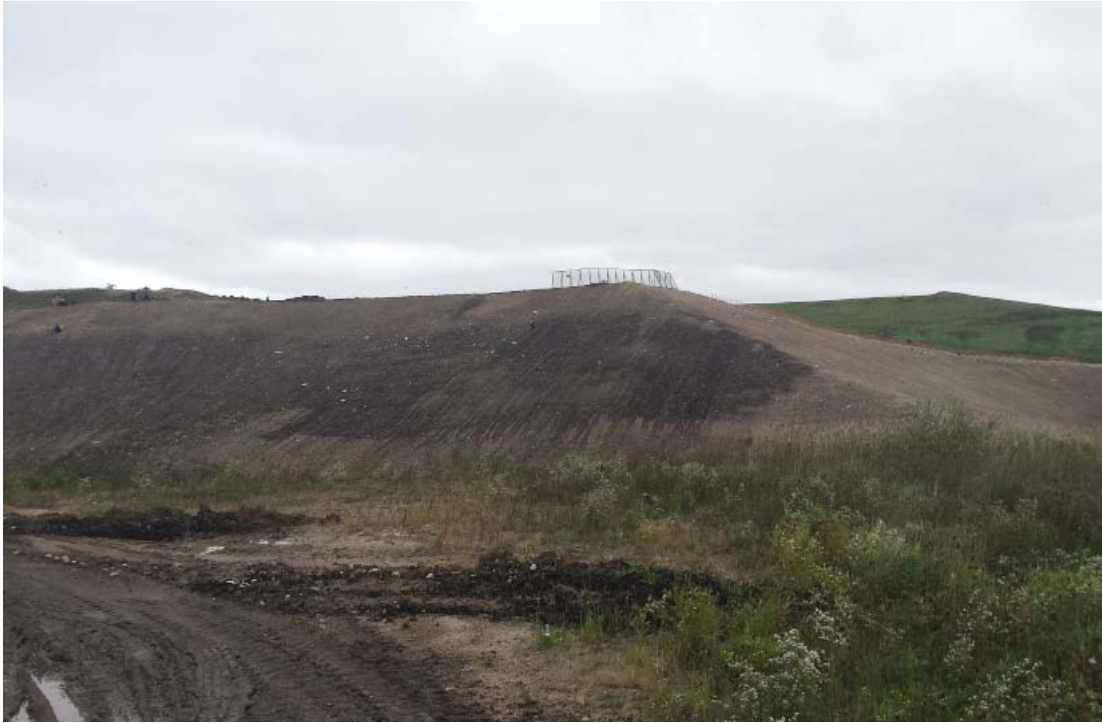
West and South slope of Phase 7
