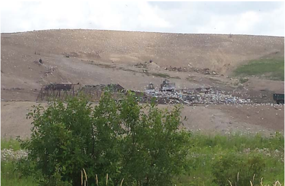
Working face viewed from West
