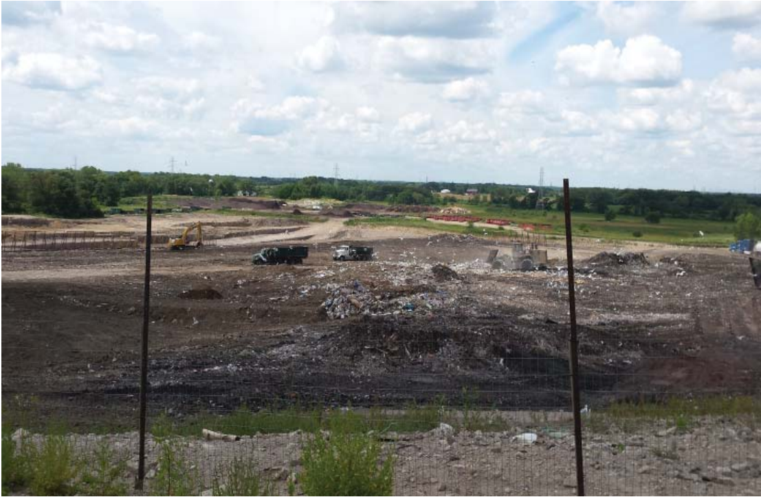
Active area viewed from Northeast
