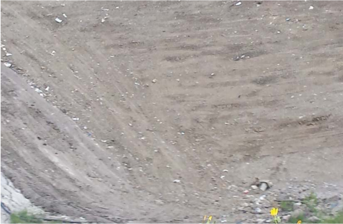
New slope over drainage layer, some flagging
