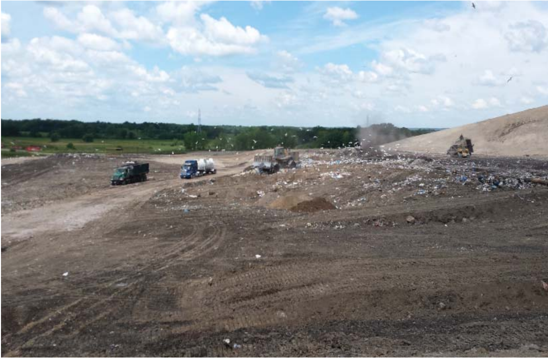
Working face viewed from East
