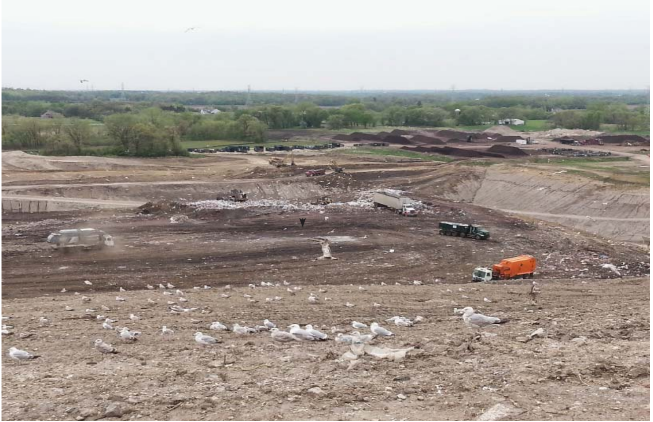
Active area viewed from the North
