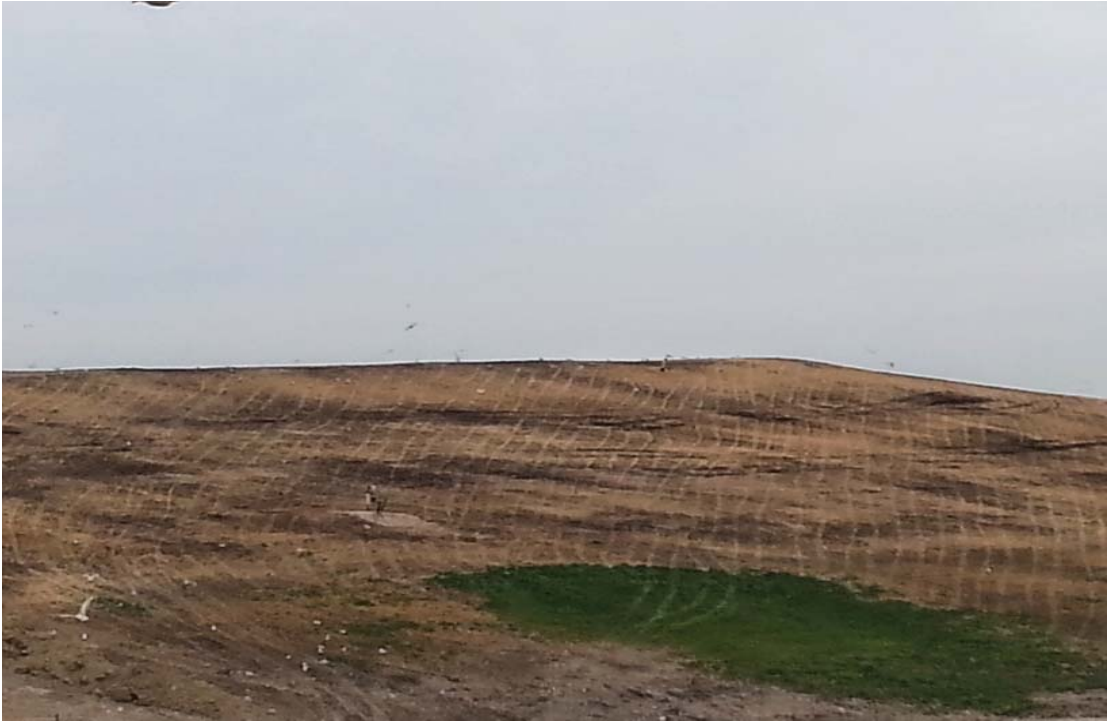
West slope of Phase 6, seeded and crimped
