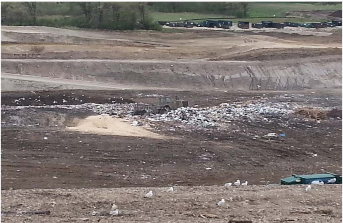
Active area viewed from the North
