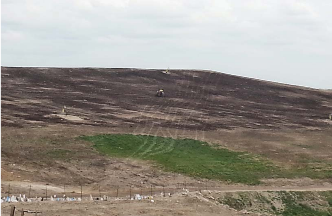
Seeding of the West slope of Phase 6
