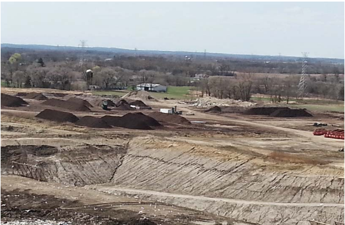
Site South of footprint, compost facility and future expansion area
