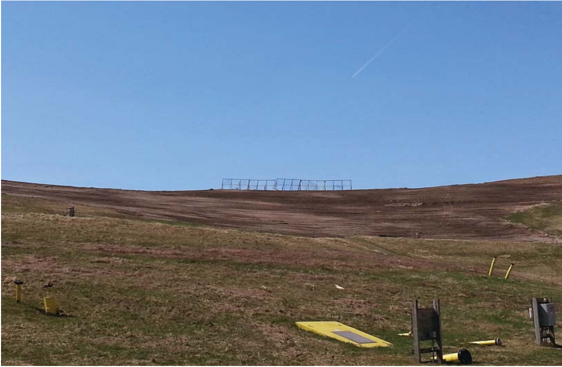
Phase 4 Northeast slope, backdragged.
