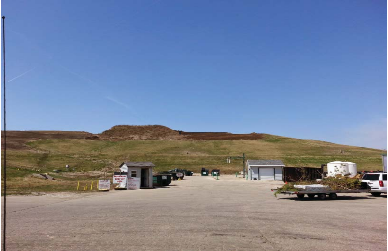
Phase 1,2,&3 top and exposed slopes dressed up
